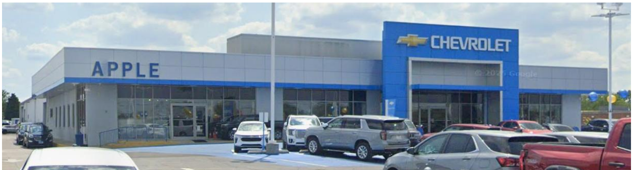
Aluminum Composite Metal panels at Apple Chevrolet (8585 W. 159 th Street)
